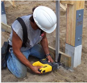
1. Drill 3/16" hole with masonry drill bit (1 1/4" deep)
