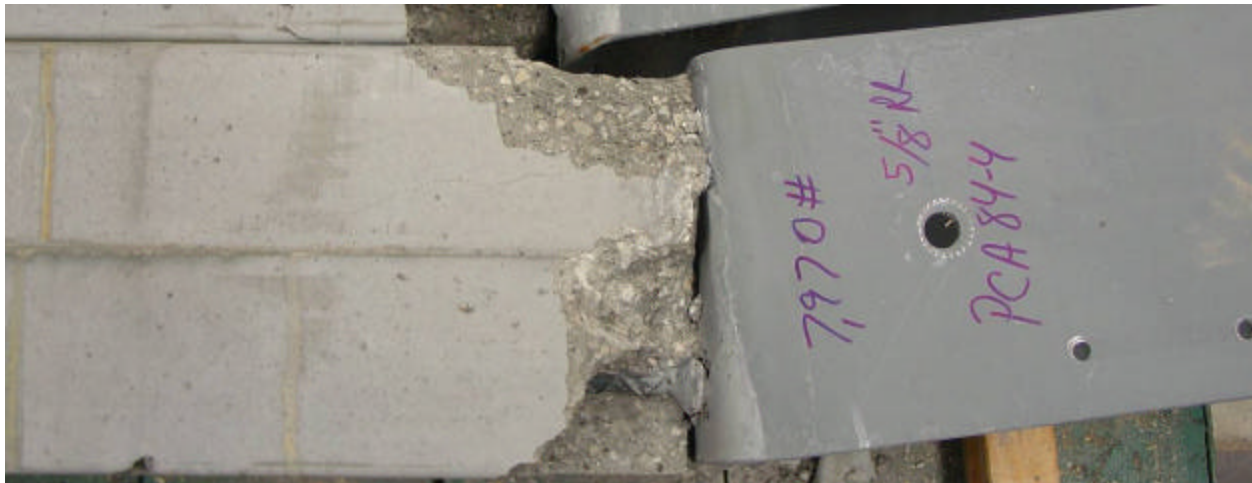
Figure B.6. Fracture of tension steel rebar connection in PC8400 replicate 4.
