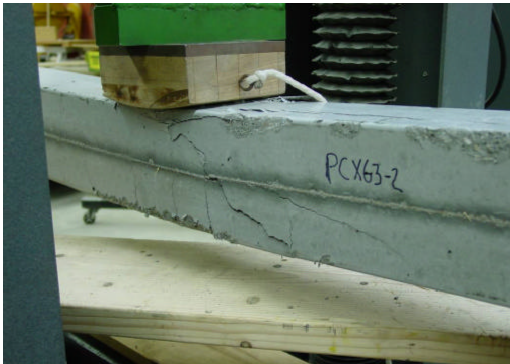
Figure A.3. Bending failure mode characteristic of all PC6300 and PC6400 series columns.
