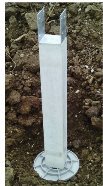
Figure 9.1: Deck Post on AG-CO Molded Plastic FootingPad
